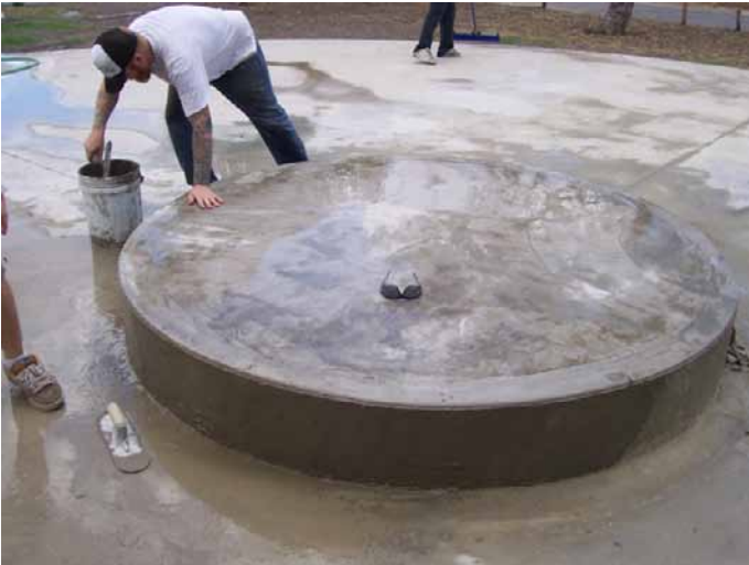
Lonestar Skateparks finishes a manual pad at Southside Lions Park in San Antonio
